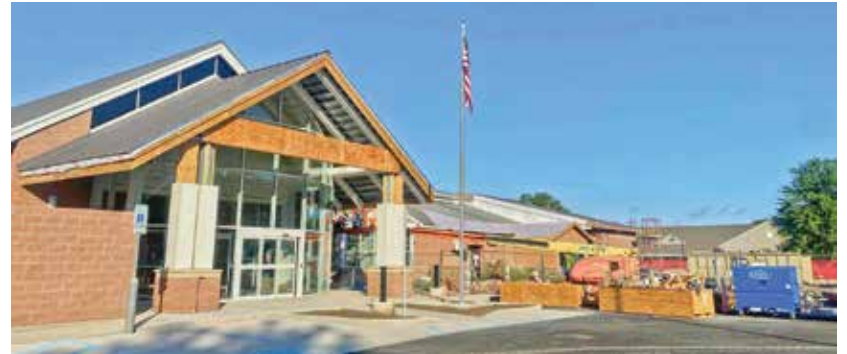
Exterior renovation continues. Completion expected later this year.
