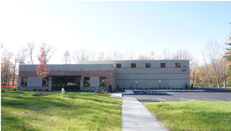
McBride Office Building
