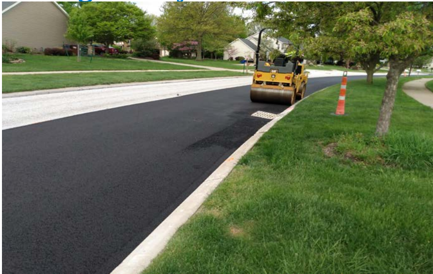
Asphalt Road Repairs
